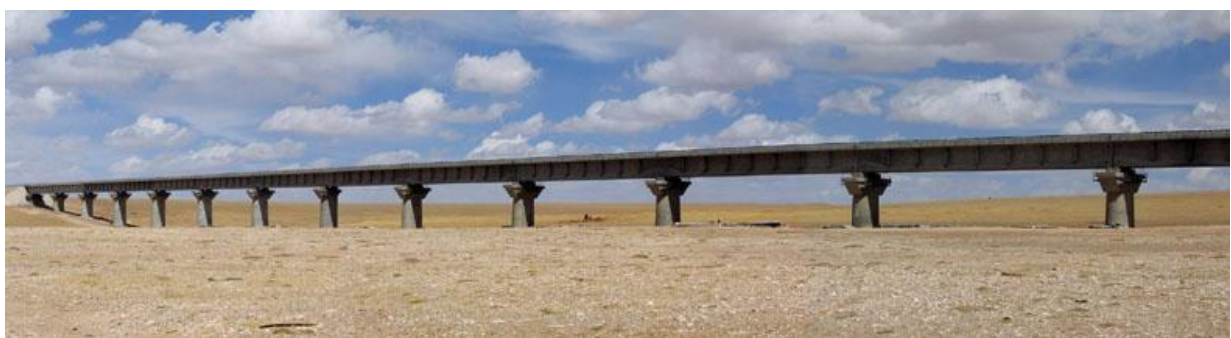
Fig 7. Wudaoliang Railroad Bridge
