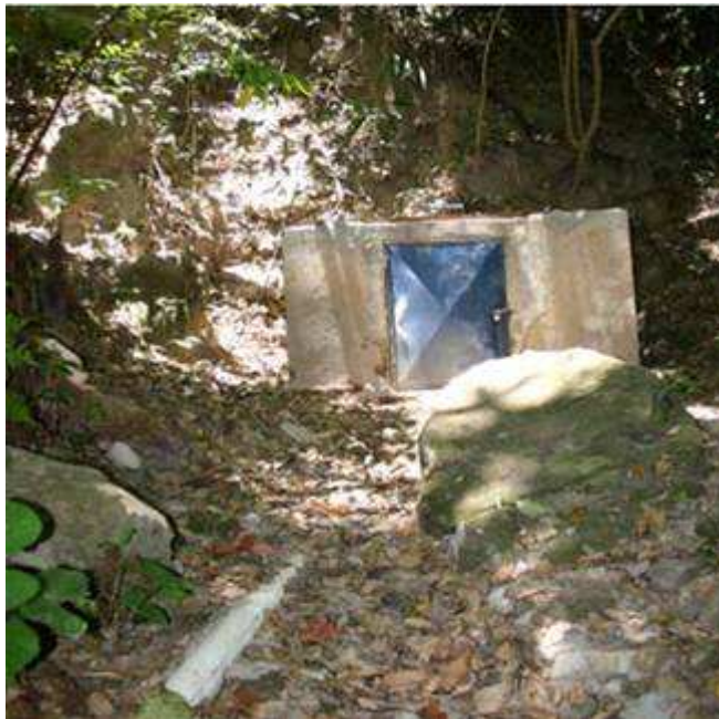
Figure 13. Concrete boxes built to control the water flow directly from the springs.
