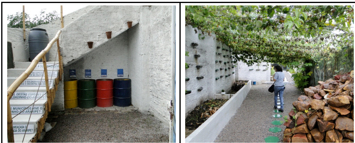
Figure 29. Various stages of construction and recuperation of the outside area in back of the ICC building to transform it into parts of the ESA. Left: recycling bins; Right: compost area, vertical garden and artificial water spring to bring a sensation of being in the humid forest.
