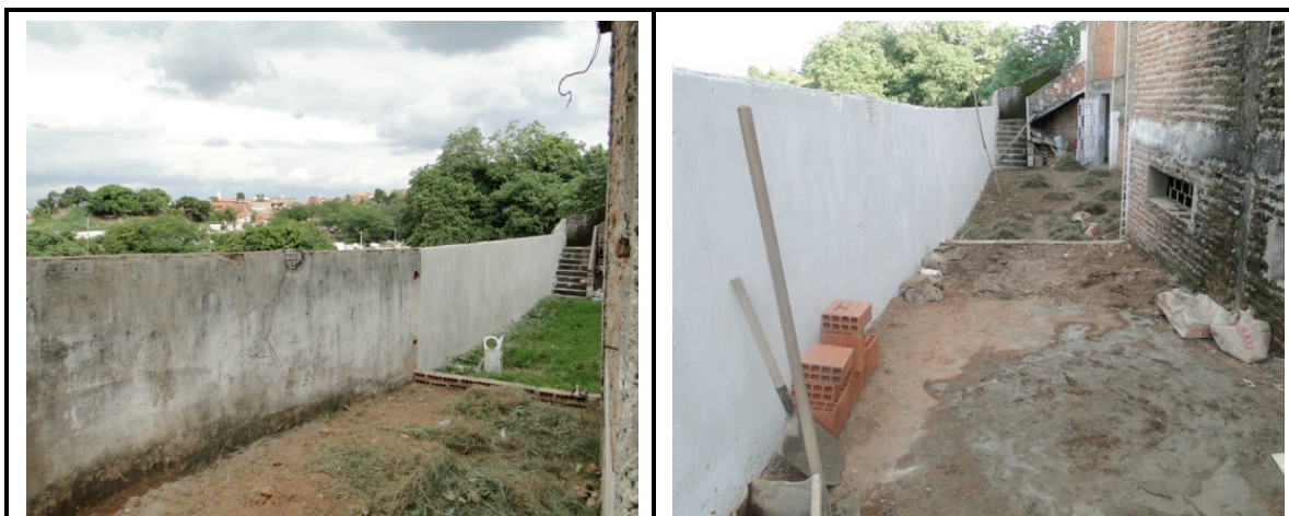
Figure 30. Early onstruction stages of the fruit drying and seed recovery beds.
